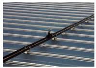
Facility has roof spraying system that uses well water to reduce the internal temperature.
